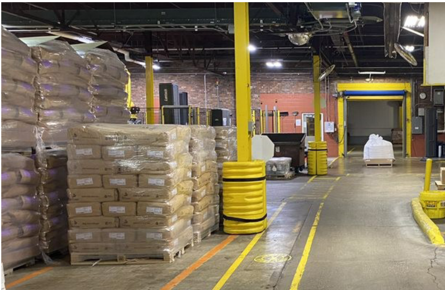
Defiance, Ohio LED lighting improvements
