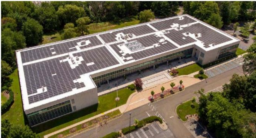
Solar panels at our Montvale, New Jersey headquarters
