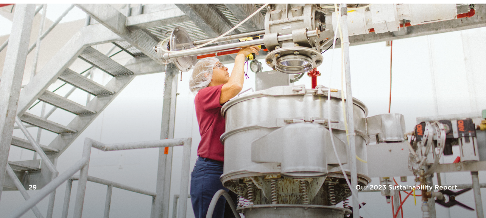
Defiance, Ohio site
