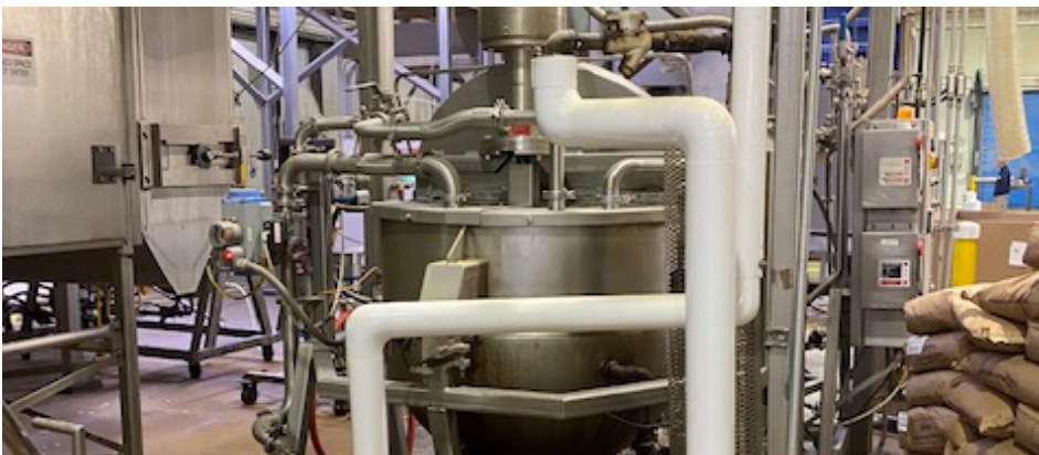
New steam and condensate system at Lincoln, Nebraska plant
