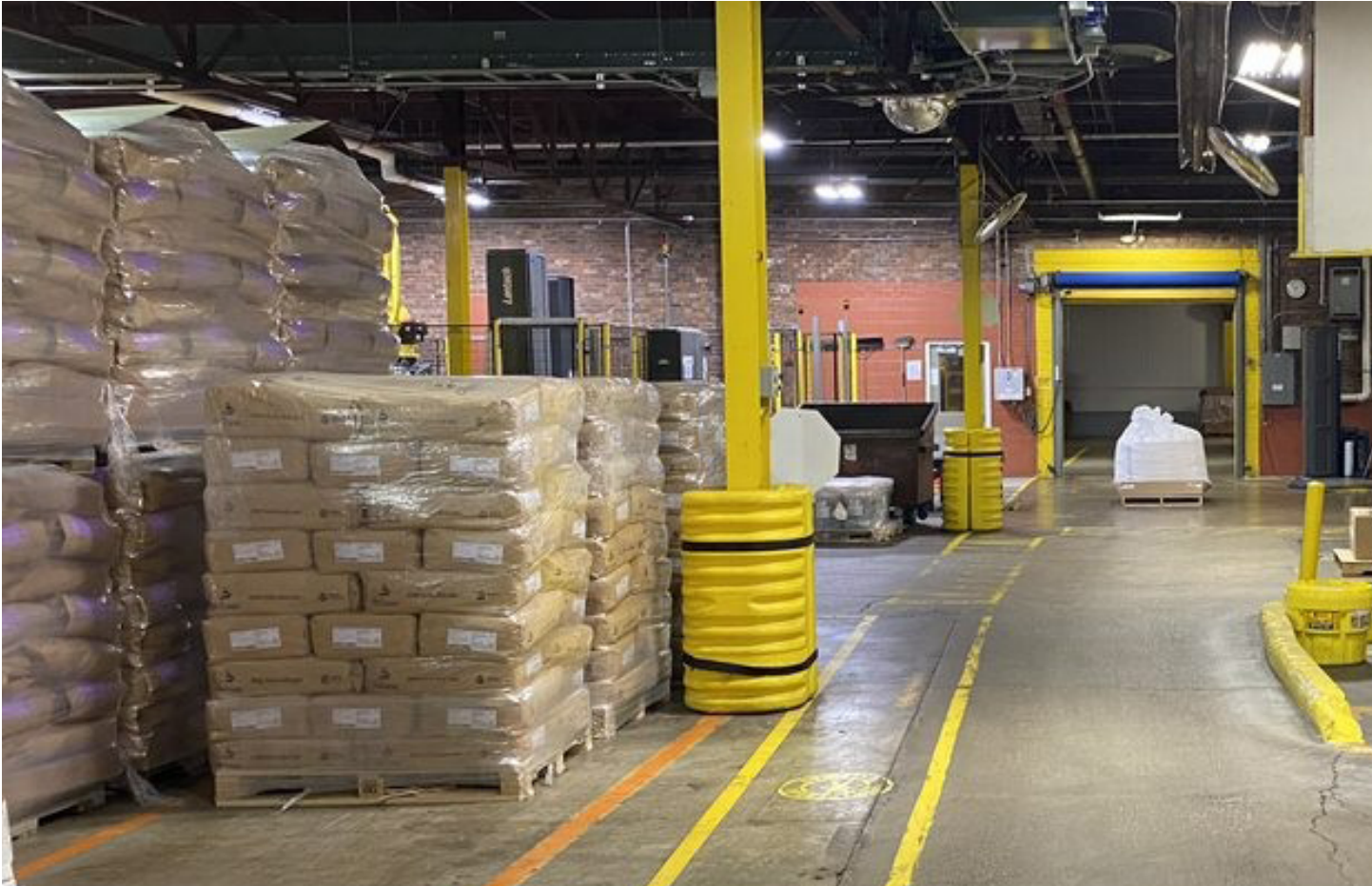
Defiance, Ohio LED lighting improvements
